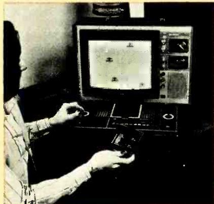
LOW-COST PROGRAMMABLE TV GAME built using new IC's from General Instrument. The game is not microprocessor based. Instead of the cartridges containing ROM memory, each cartridge contains a dedicated game IC.
